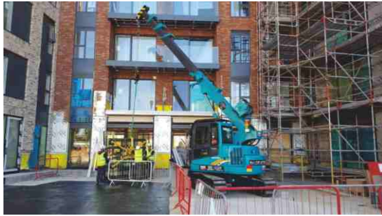
SWTC5在英国施工 SWTC5 Construction In British
