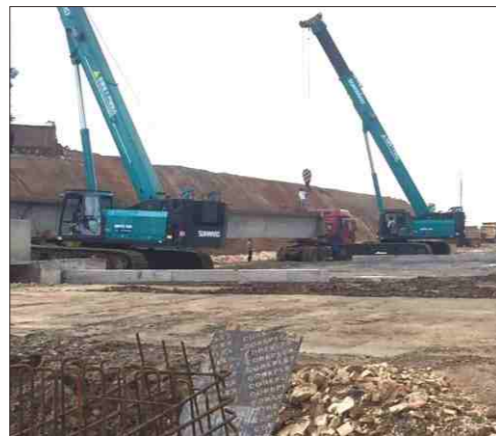
SWTC75在云南省曲靖绕城高速施工 SWTC75 Yunnan province Qujing City Expressway Construction
