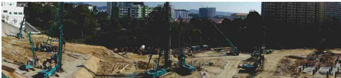
SWTC35、SWTC55在马来西亚与山河智能产品共同群体作业 SWTC35/SWTC55 Group Working With Sunward' Products In Malaysia
