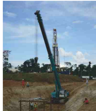
SWTC35在秘鲁施工工地狭小地带作业 SWTC35 Working In Narrow Area In Peru
